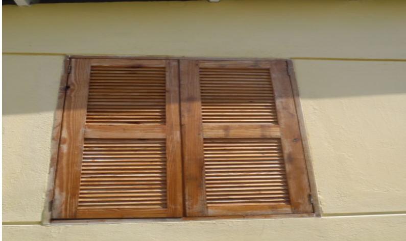
Shutters on house at Caracol-EKAM lack a second coat of varnish to prevent wood damage. (Photo by RIG/San Salvador, July 1, 2013)
