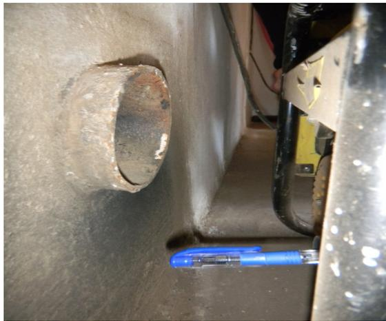
**The blue pen protrudes from the generator's exhaust pipe to illustrate that the pipe does not align with the wall penetration on the left. (OIG photograph, September 9, 2011)**
